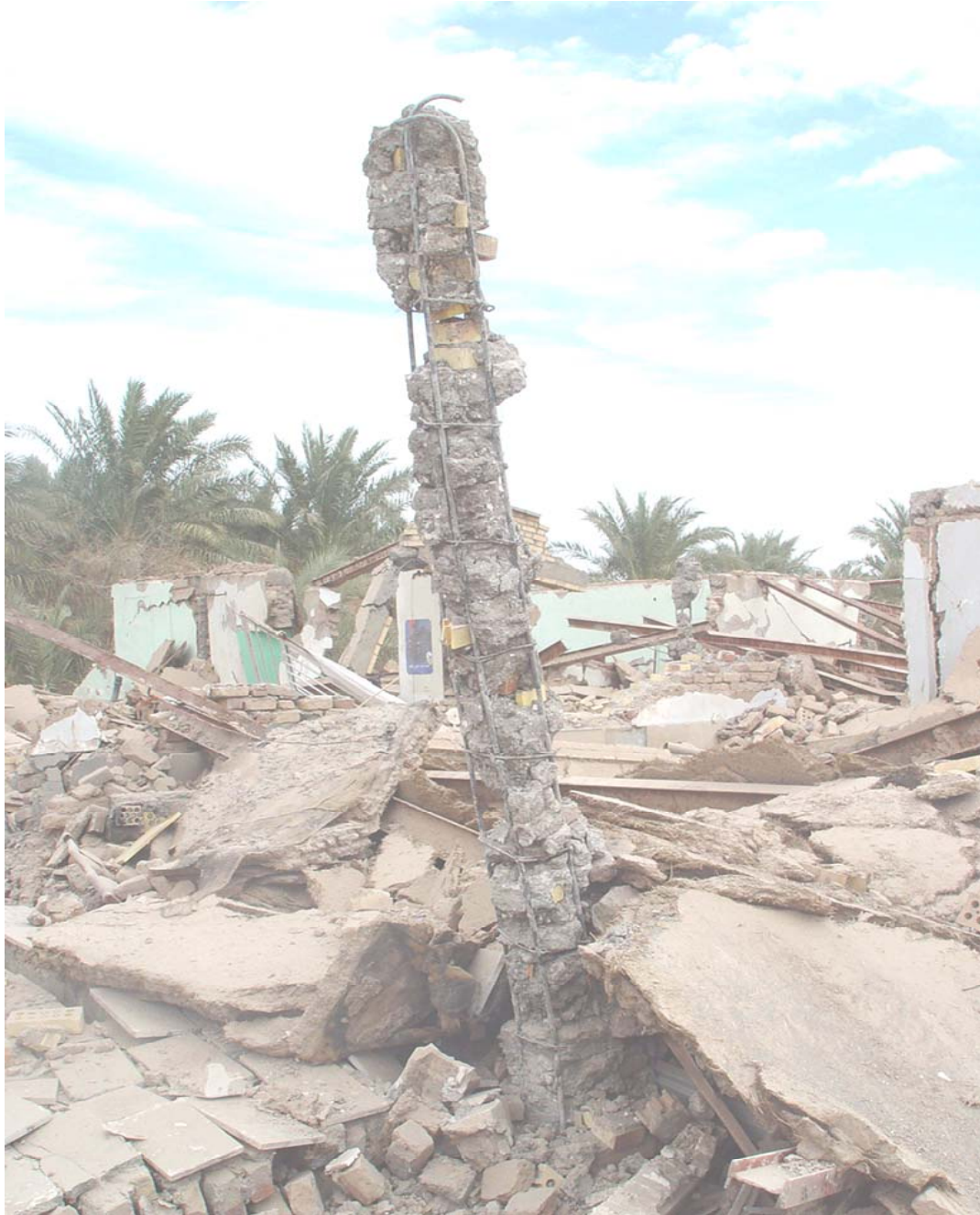
Mixing of concrete and brick in vertical ties.
