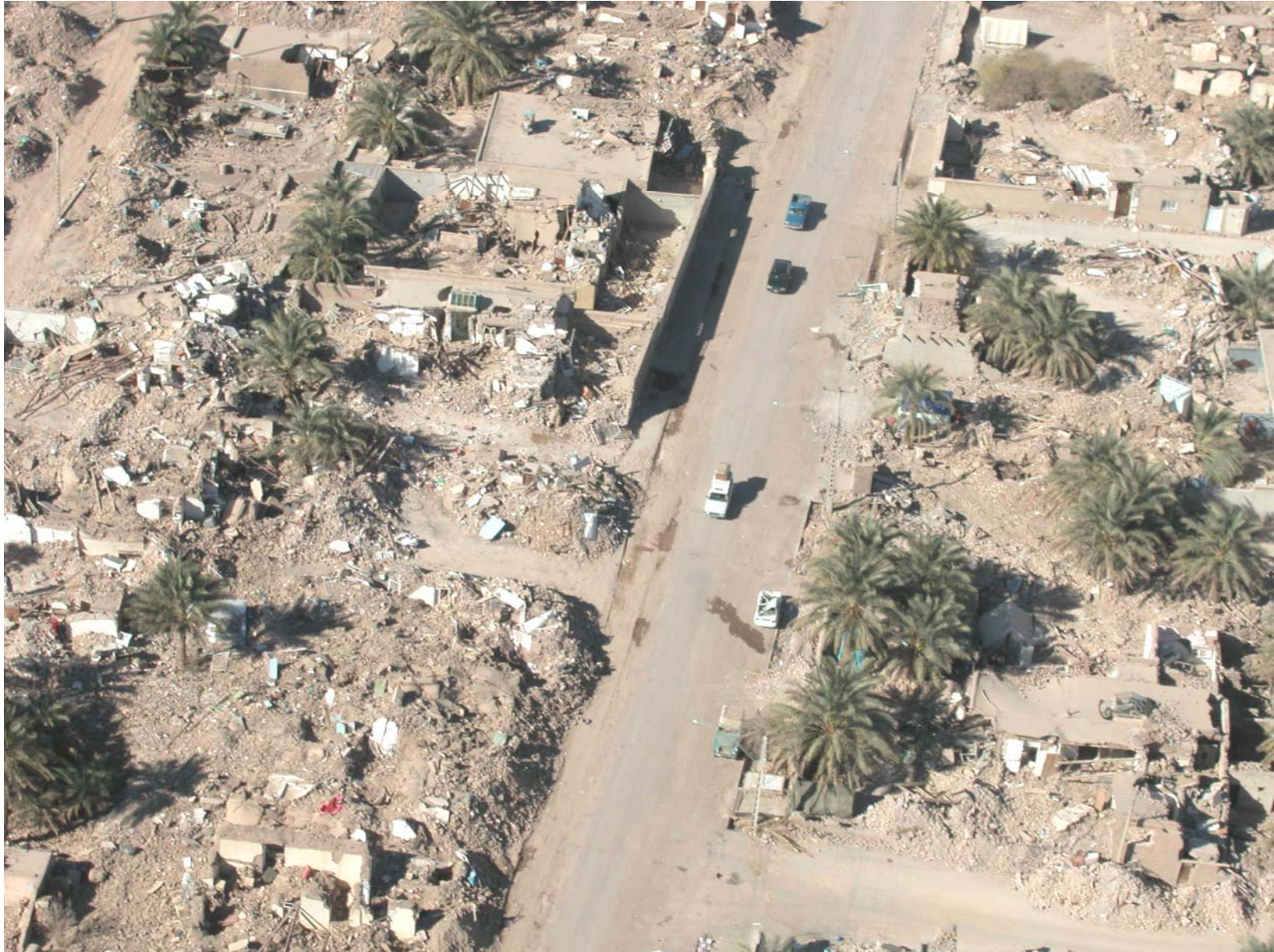
Aerial view of complete destruction of adobe dwellings the Bam earthquake.
