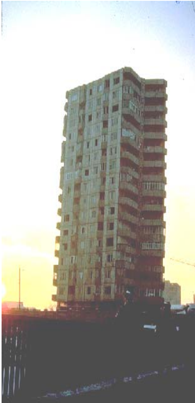
16-story lift-slab concrete building in Leninakan. The building is leaning about 1 meter to the right and is a total loss due to a general failure of the cast-in-place concrete shear core at the ground level.
